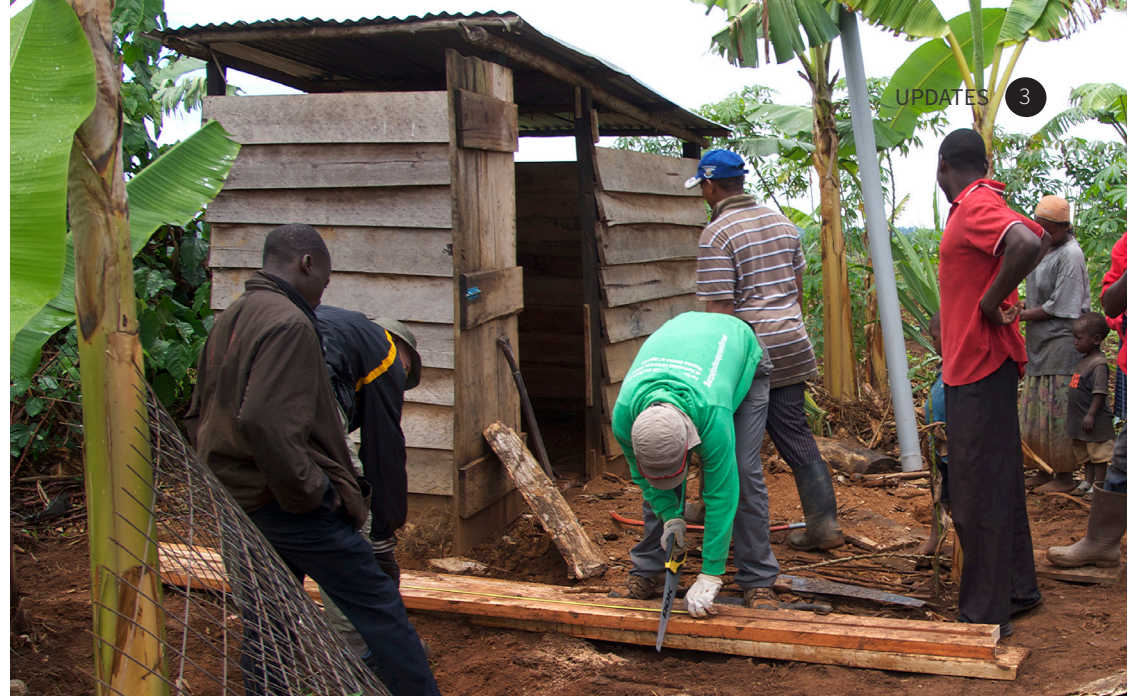
Repairs to the latrine at Maama Rose's.
